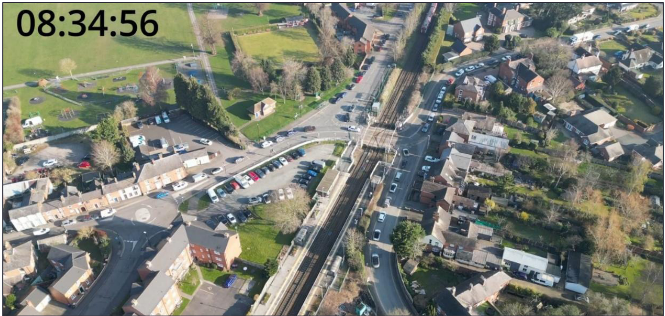
Figure 6.1 Level Crossing – AM Peak Before Opening
